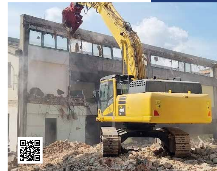
Bologna, building demolition intervention
