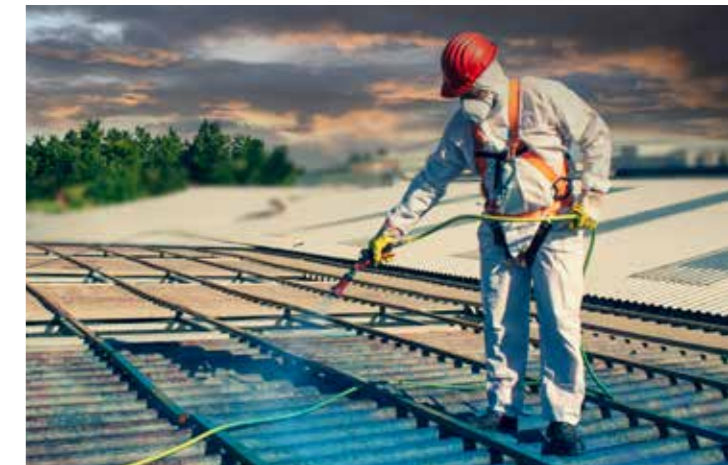
Remediation through conservative encapsulation of asbestos cement roofing
