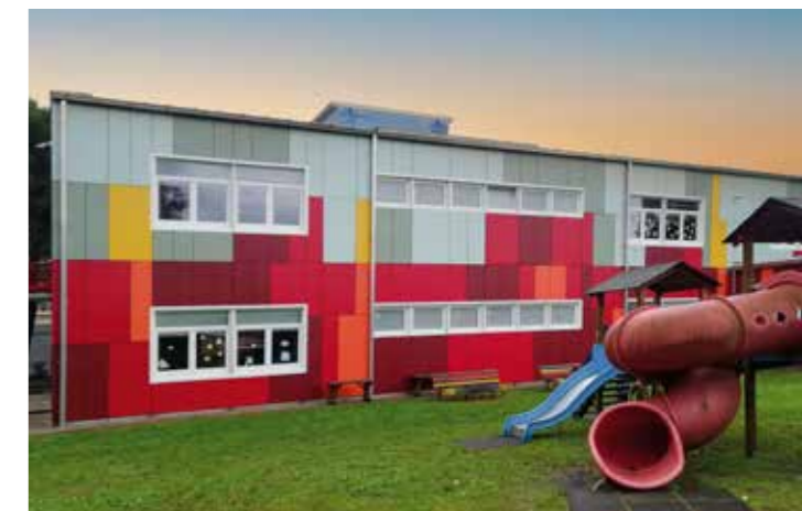
Sestri Levante (GE), eco-efficiency and energy consumption reduction interventions at the school complex
