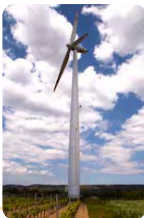
The renewable energy and energy-saving sector was established.
