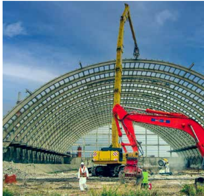
Crotone, Syndial SpA, Building Demolition Intervention
