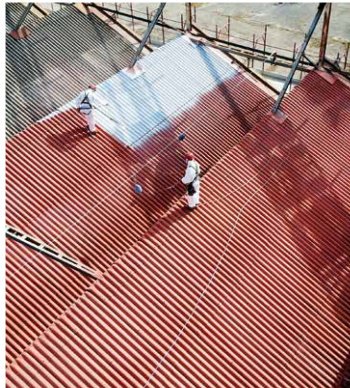
Bari, Caserma Rossani, remediation through conservative encapsulation of asbestos cement roofing.
