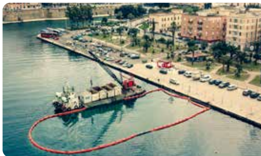
Removal of anthropogenic materials from the seabed of the Mar Piccolo in Taranto
